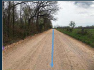
BEFORE: Water flowing unimpeded down roadbed, picking up velocity and sediment, causing EXTREME ditch erosion and sediment pollution into Little Osage Creek.
