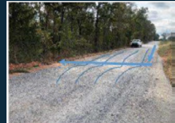
AFTER: Broad based dip intercepts approximately 1,500 feet of flow and directs it into wooded area to be dissipated.
