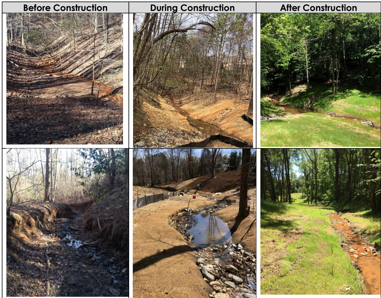
Figure 6. Before and after conditions of the RiverRun stream restoration that was constructed in place of a historic dry detention basin.
