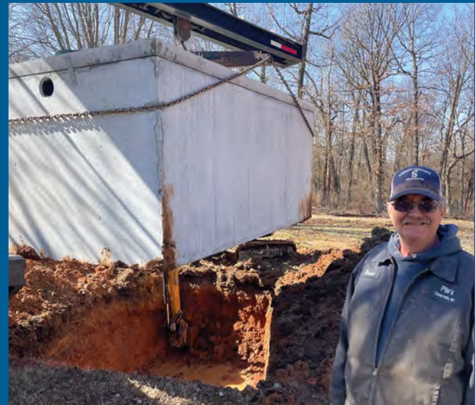
Pyle's Concrete sets a 1500 gallon tank in Lowell.
