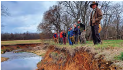
Partners visit a highly degraded site on Wildcat Creek in planning out restoration work.
