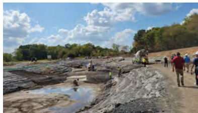
WOKA whitewater park under construction in September 2022.
