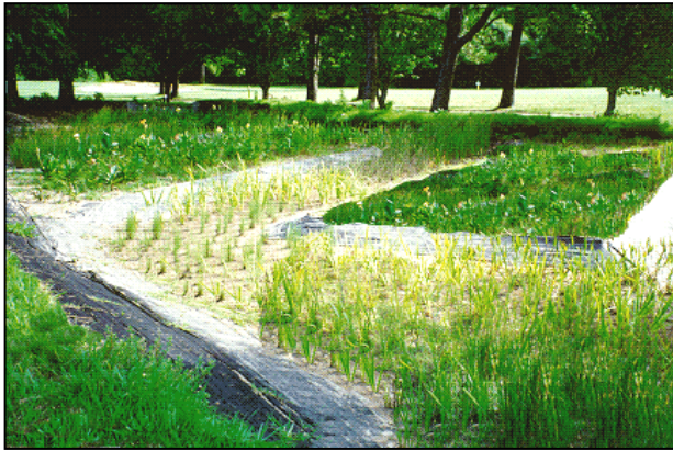
Newly Constructed Shallow Wetland
