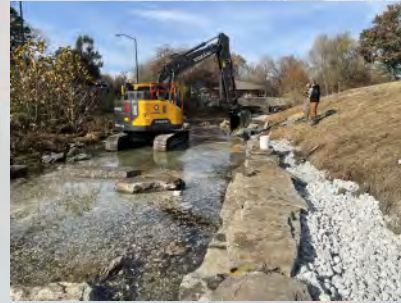
Streambank stabilization on Sager Creek
