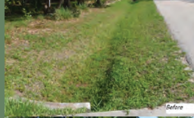
A ditch re-vegetated to treat stormwater Photo by Phillippi Group
