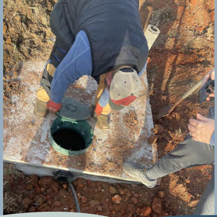
Porter Backhoe sets and tests a new 1000 gallon tank for leaks.
