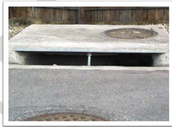
(b) CDOT Type R curb opening inlet
