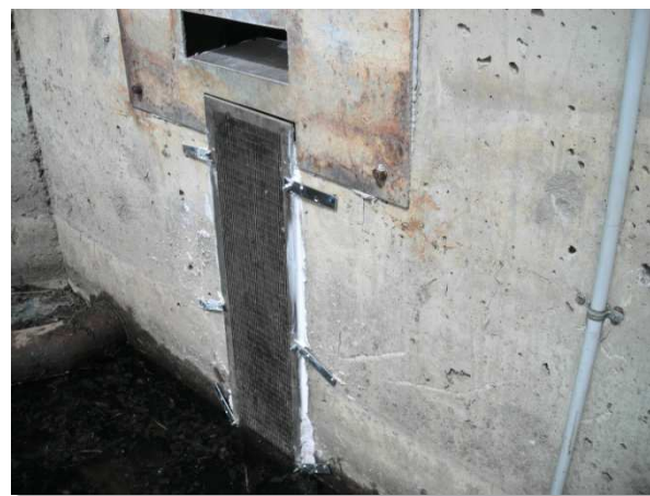
Photograph OS-3. Trash rack after repair.
