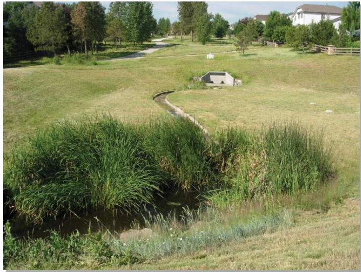
Photograph EDB-1: This EDB includes a concrete trickle channel and a micropool with a concrete bottom and grouted boulder sideslopes. The vegetation growing in the sediment of the micropool adds to the natural look of this facility and ties into the surrounding landscape.
