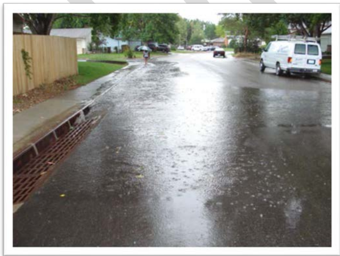
Photograph 3.4.2-1. Weir performance decay can be observed in this picture as flow appears to enter only the first two inlets while exceeding the height of the upstream curb.
