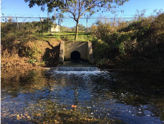
Figure 17. Wastewater effluent in Sager Creek.
