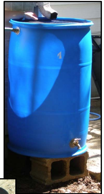
Bulkhead Tank Fitting
