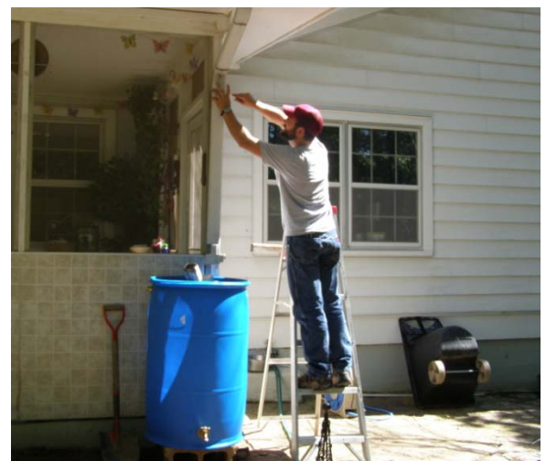
Reconnect the elbow and downspout to the gutter.
