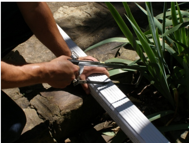
Remove downspout and cut it at the appropriate length.
