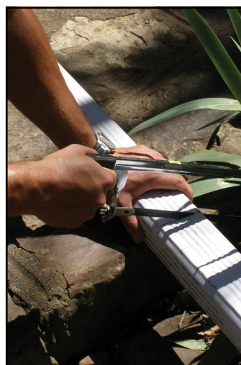
Making the gutter cut for new elbow placement.
